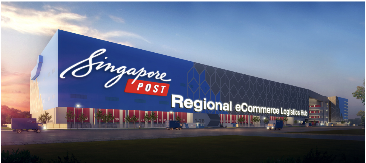
Artist's impression of façade of SingPost's eCommerce Logistics Hub in Tampines LogisPark
