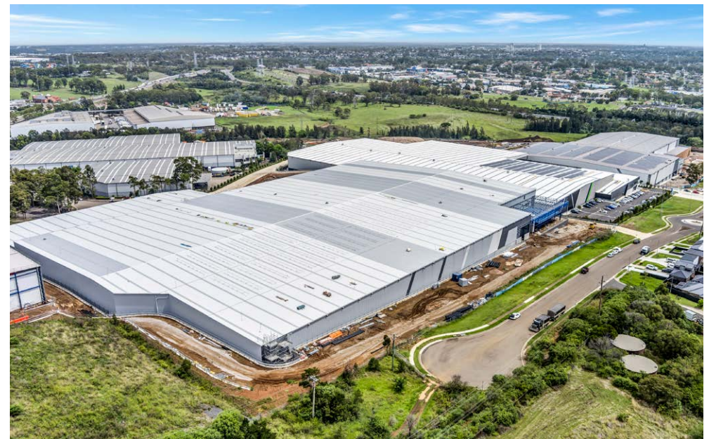
> CouriersPlease Pemulwuy depot scheduled for completion in mid-2024 designed to Green Star Standards
